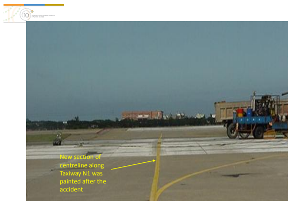
Figure 13 – A new section of Taxiway N1 centreline marking added and Runway 05R threshold markings (piano keys) being removed soon after the accident
