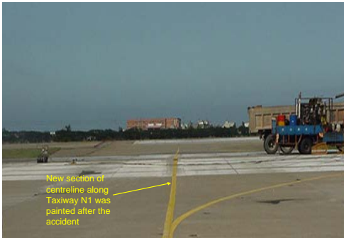
Figure 13 – A new section of Taxiway N1 centreline marking added and Runway 05R threshold markings (piano keys) being removed soon after the accident
